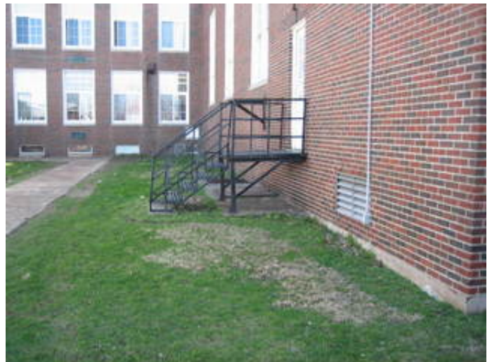
Exterior egress stair
