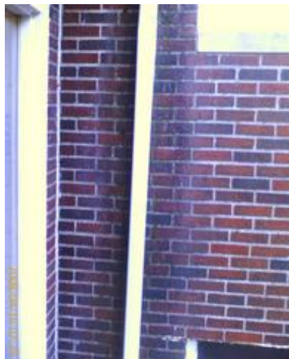
Typical exterior wall condition
