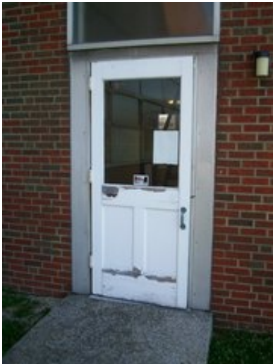
Typical exterior door
