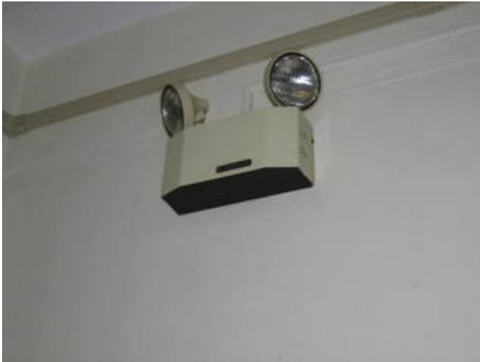
Corridor mounted emergency lighting
