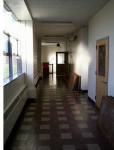
VAT in corridor of 1975 addition
