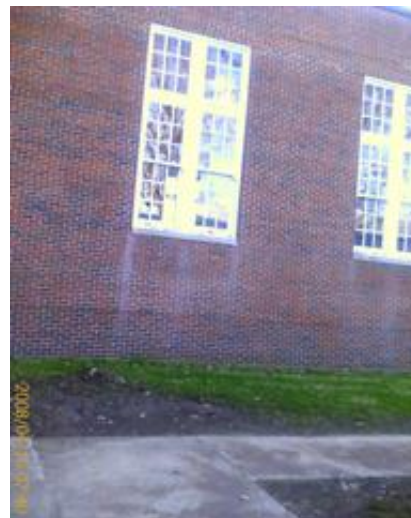
Typical exterior wall condition
