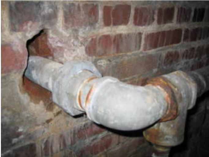
Water service entry
