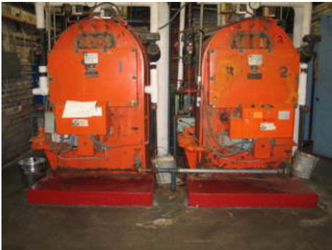
Natural gas steam boilers
