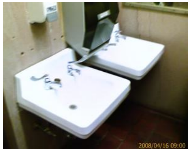
Typical fixture condition
