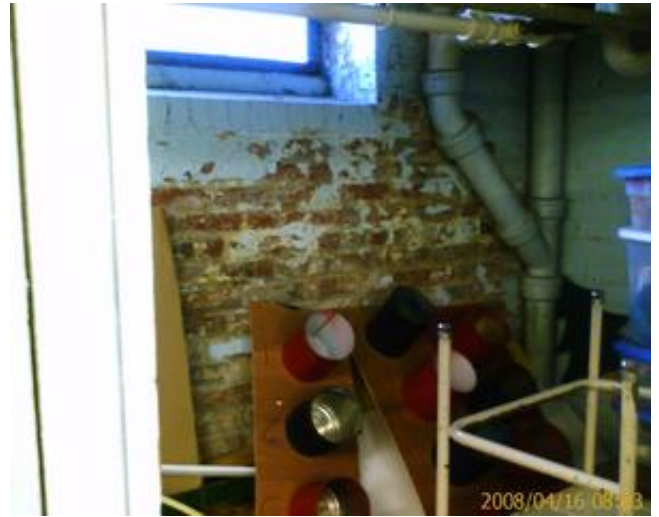
Typical masonry foundation wall
