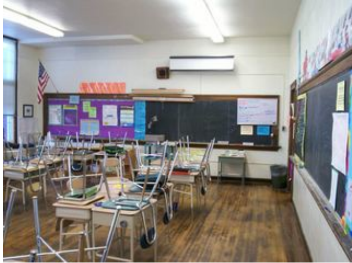
Typical classroom finishes in the original construction
