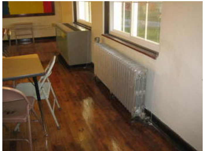
Classroom unit ventilator and radiator
