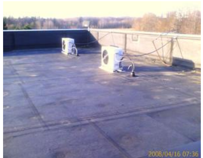
Typical EPDM roofing system
