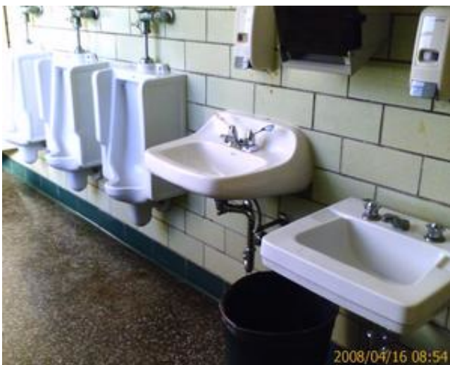
Typical fixture condition
