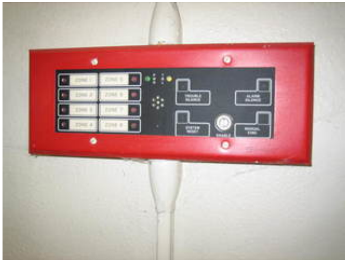
Fire alarm annunciator panel
