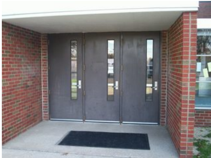
Entrance door in the 1975 addition
