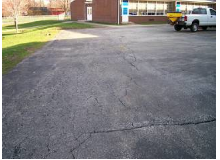
Asphalt pavement in poor condition
