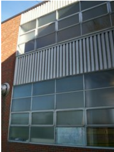
Typical windows in the 1975 addition
