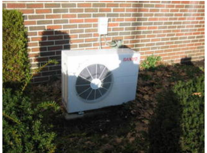
Pad mounted condensing unit
