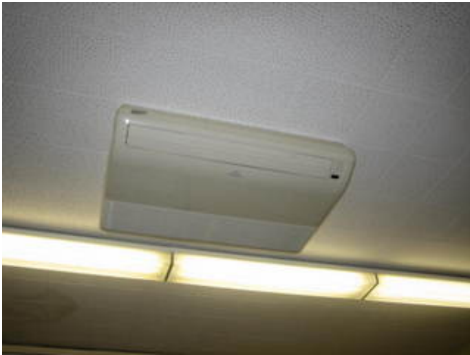
Ceiling mounted air conditioning unit
