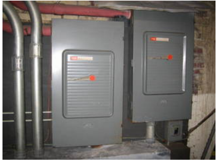
Main electrical disconnects
