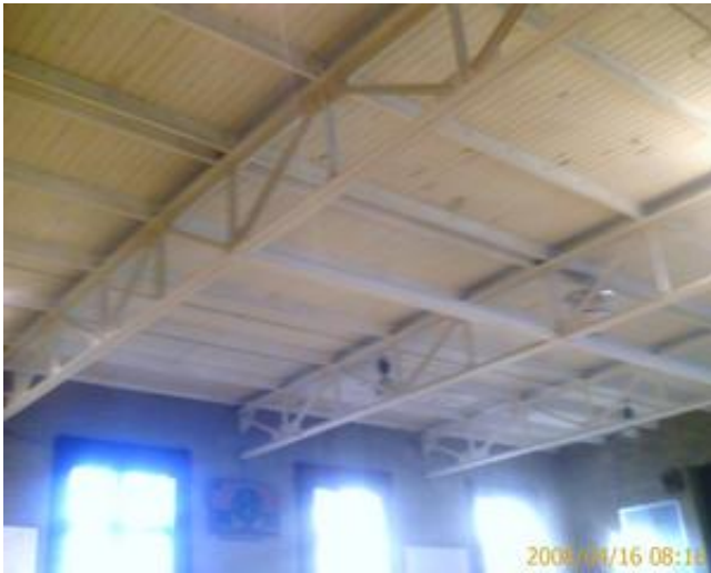
Typical wood roof deck
