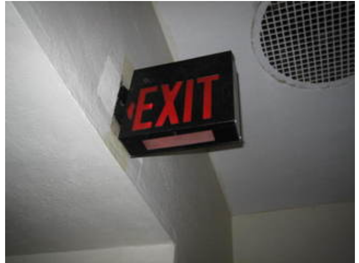
Corridor mounted exit signage
