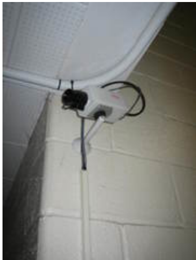
Corridor mounted security camera
