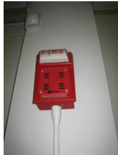
Corridor mounted horn/strobe device
