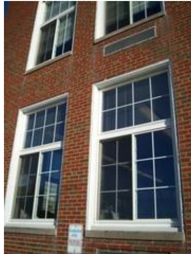
Vinyl windows in the original construction and 1956 addition
